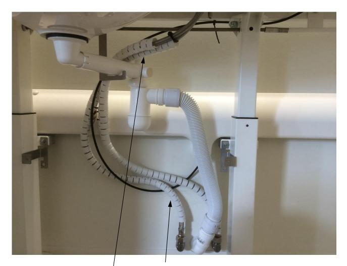
Cable binder mounted on water hose
